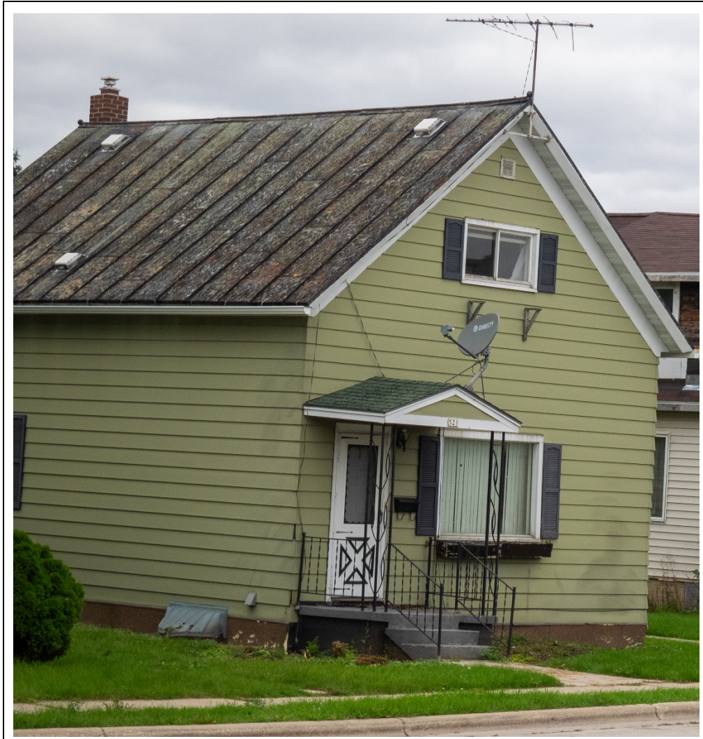
521 Fifth St.- appears to be reasonably well maintained but starting to show some deterioration.
