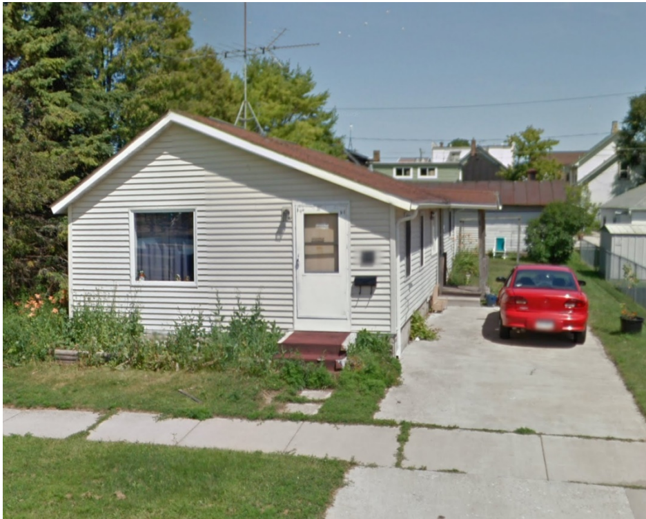
516 Sixth St.- appears to be well maintained.
