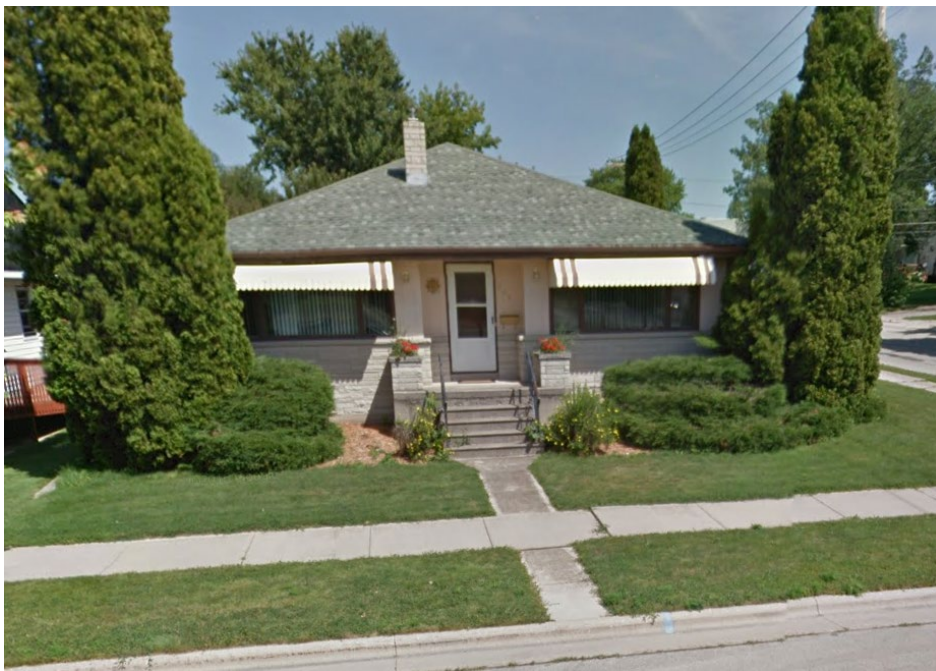
528 Sixth St.- appears to be well maintained.
