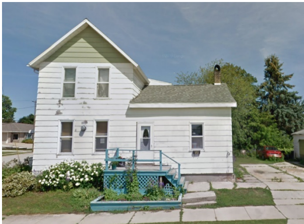
520 Steele St. – top photo from Oct. 2019, bottom photo by Google Maps from July 2013, showing continued exterior deterioration.
