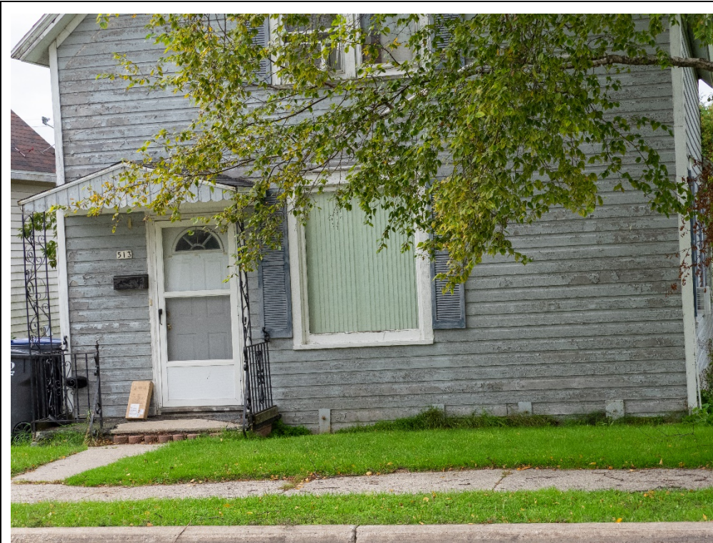
513 Fifth St.-siding and trim need paint, overgrown tree and trees growing next to foundation on side of house.
